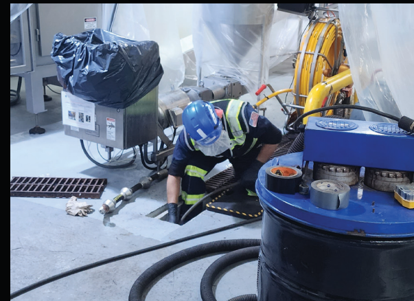
Fig. 2 Pipe being prepared for lining
