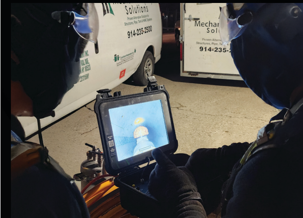
Fig. 1 Video inspection of pipe
