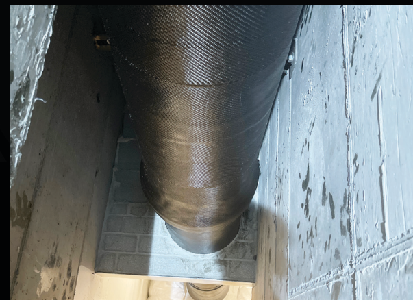
Fig. 3 Through-wall penetration after installation
