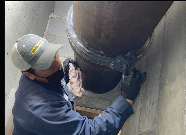
Fig. 1 Bell and spigot joint smoothed with repair putty
