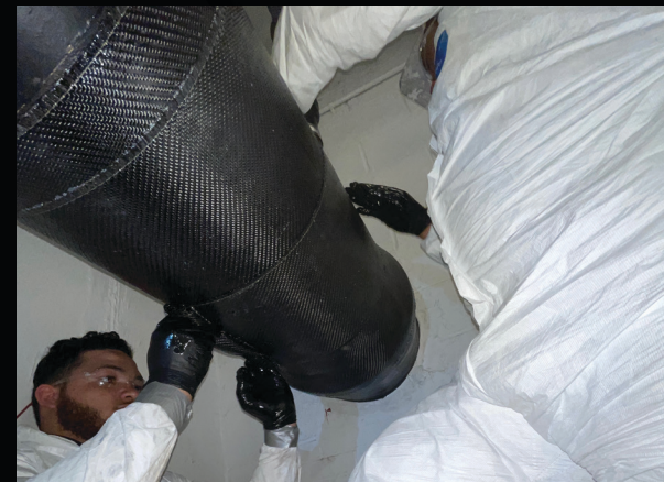
Fig. 2 Composite wrap installation
