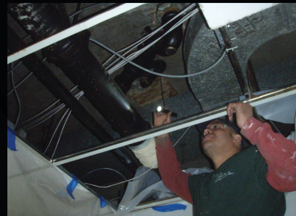
Fig. 1 Inspection of piping
