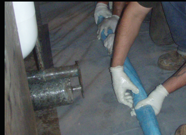
Fig. 2 Preparation of CIPP liner
